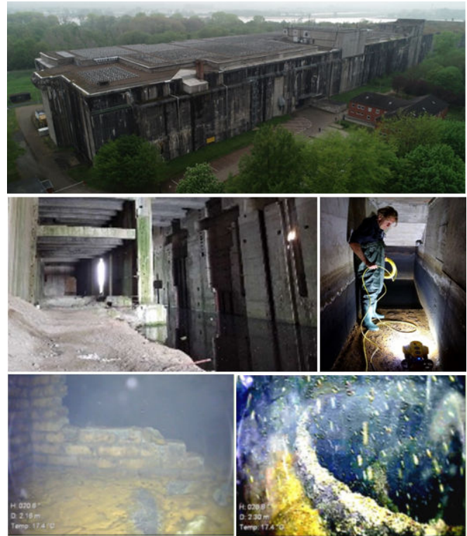
Fig. 1: The WWII submarine-bunker Valentin (top) is mapped by air-, ground-, and underwater-robots as part of a project on the digitization of cultural heritage [7]. Especially the flooded parts of the bunker (center) - including maze-like basements - are of interest to historians as there are differences to the original construction plans, e.g., unexpected walls or structures (bottom).
